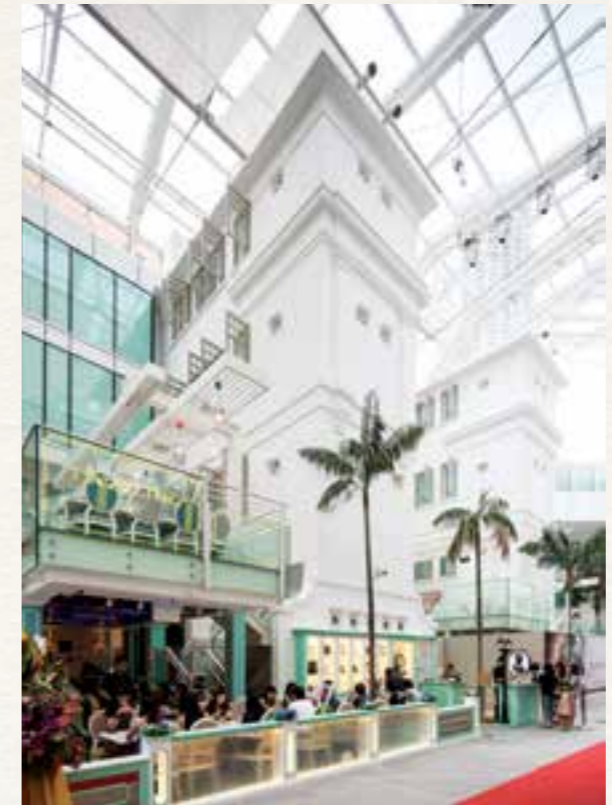
Capitol Singapore's design maximises daylight usage as a natural light source to reduce lighting requirements.
