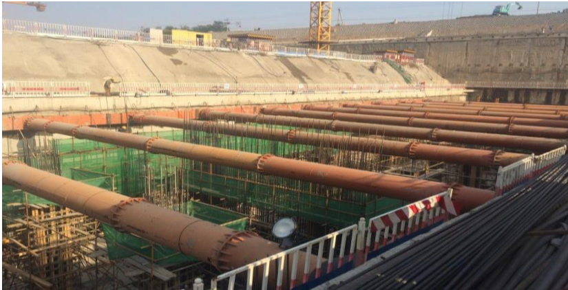
Extensive construction work for Subway (Line S6) underway.
