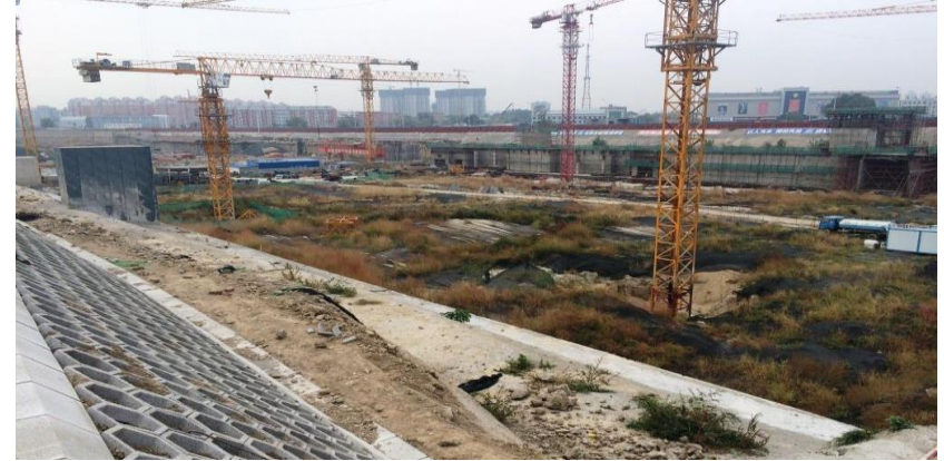
Site construction activities are in progress.
