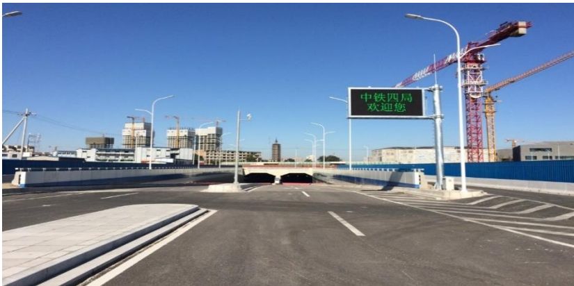
Dong Guan Avenue, to the West of the integrated development, is ready to be opened to traffic.
