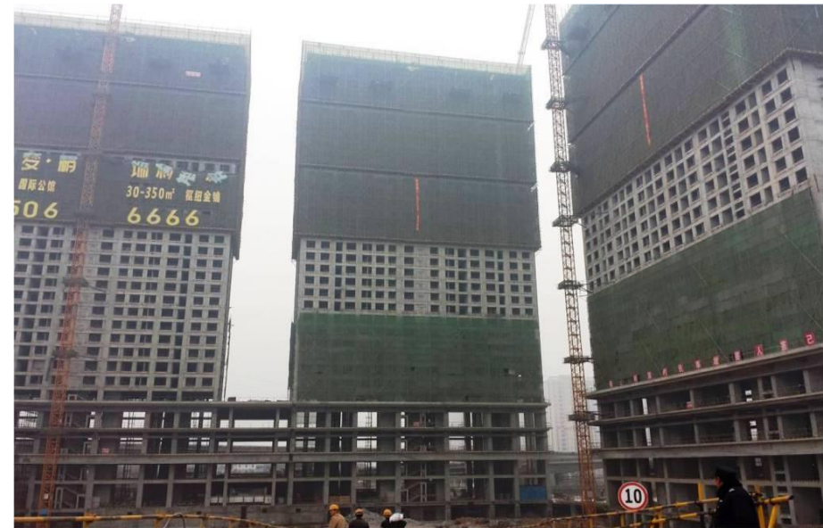
On-Site Photo – 3 Blocks on D2
